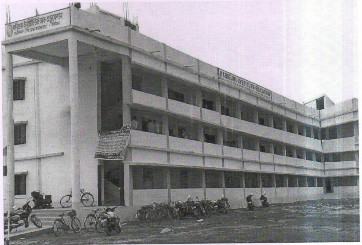
Rear view of the building
