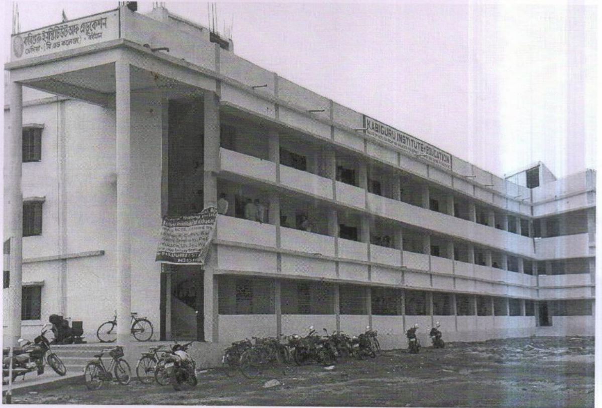
Front view of the Building
